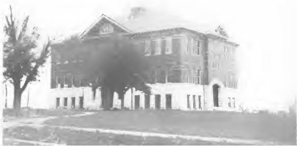
HIGH SCHOOL BUILDING, AUGUSTA, KANS.
